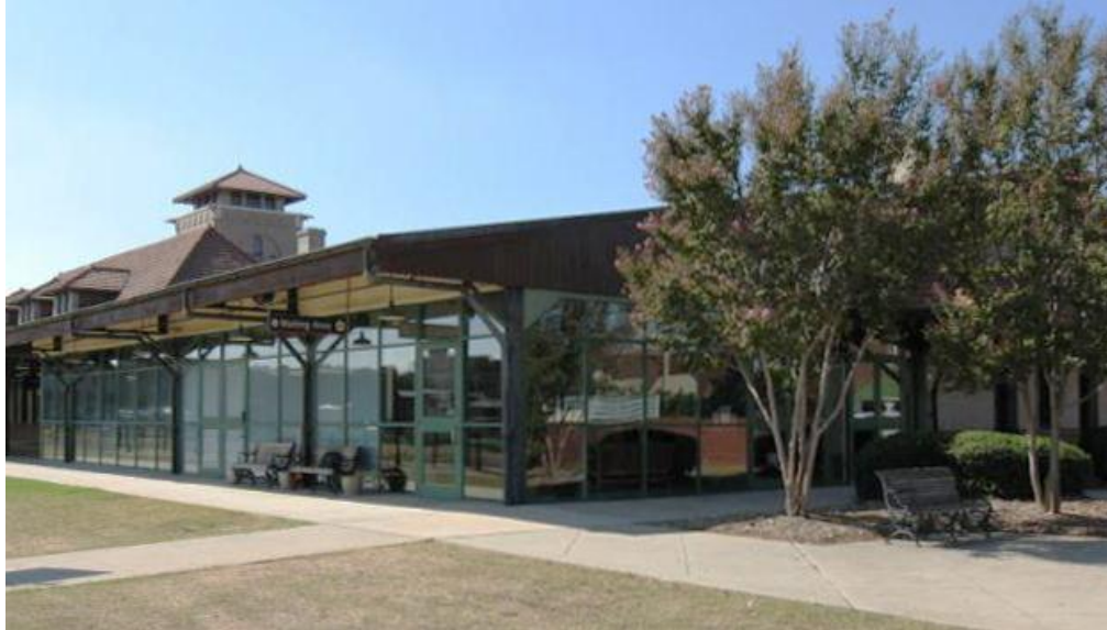
Space underneath the trackside canopy was enclosed with glass to create a modern waiting room; the historic waiting room is rented out for special events to raise revenue for building maintenance.
